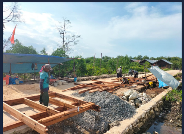
Wall Frame Manufacturing
