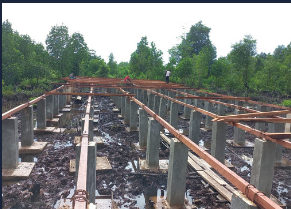
Installation of The Lower Beam
