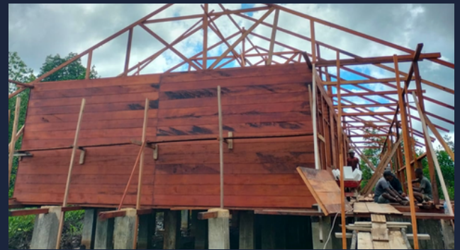
Wall Board Finishing
