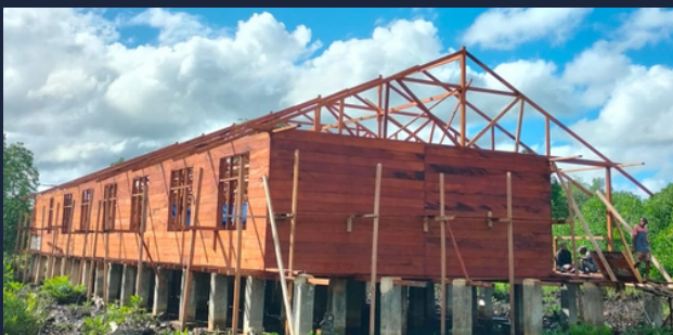
Roof Frame Installation
