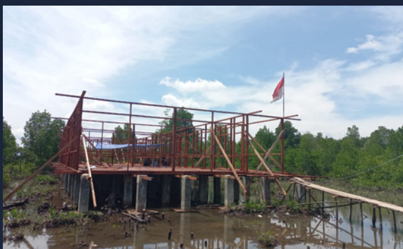
Building Frame Manufacturing
