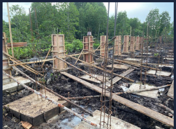
Foundation Making - Pole Cast
