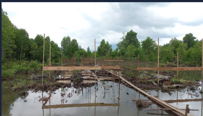
Foundation Making - Bottom Cast
